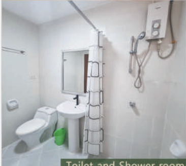
Toilet and Shower room
